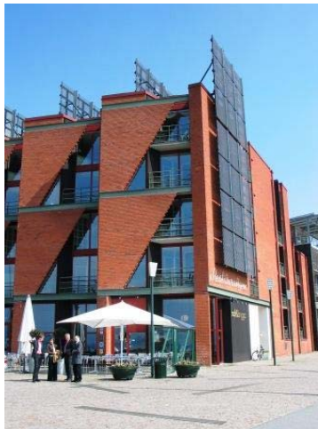
[examples of solar water heating at western harbour, Malmö and Kronsberg-Hannover]
